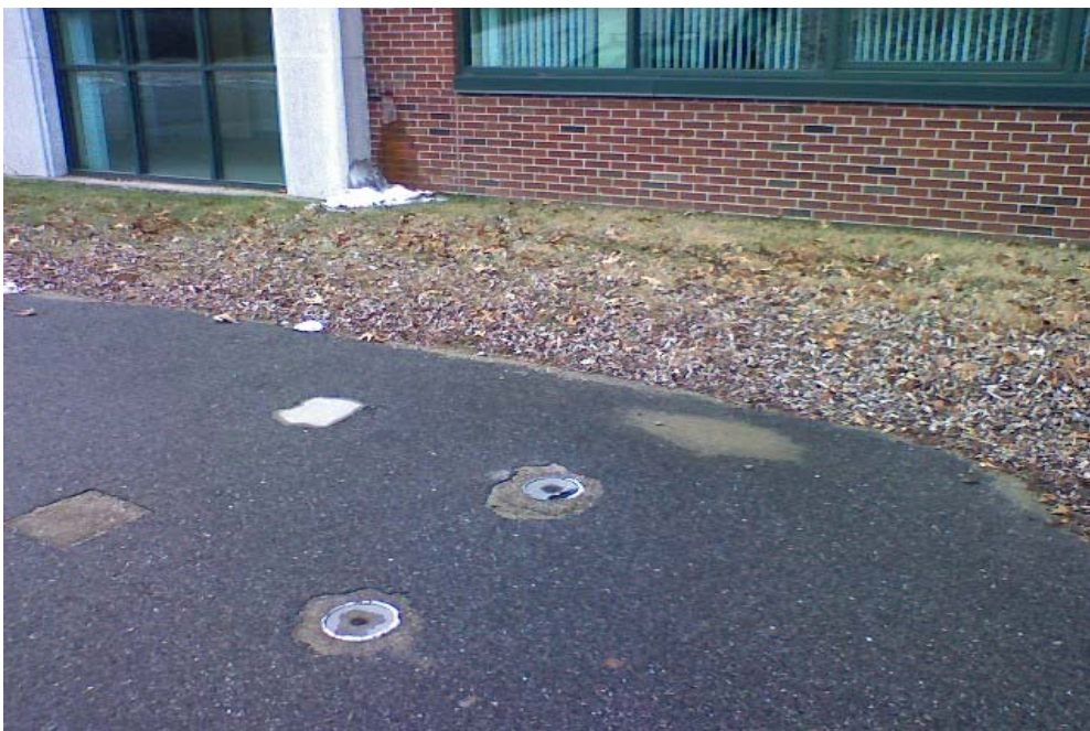
Photograph 4 - MW-40 & MW-40S with Standpipe in Background (23 January 2007)
